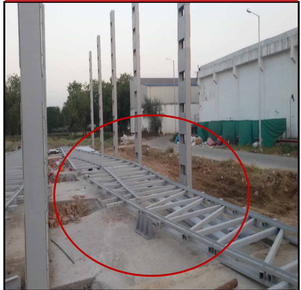
4. Truss Assembly
